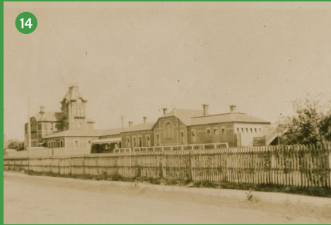
The Benalla Railway station.
